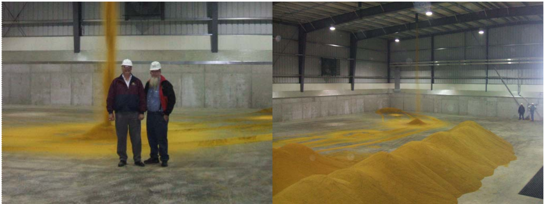
Jim Leiting and Raymond E. Defenbaugh enjoy the first DDGS flowing in the new building from the doubling project.
