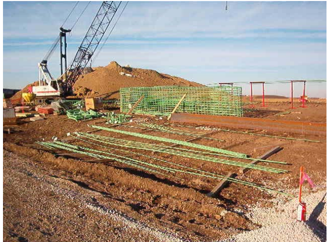
Galva—Rebar for the bridge.
