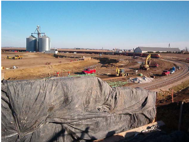
Galva—View from south of the bridge.
