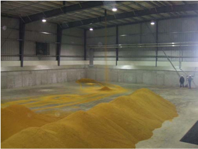
The first DDGS being produced in the new building.
