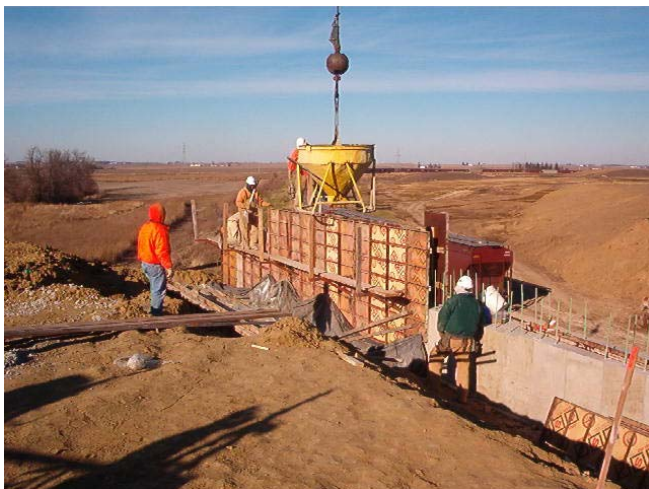
Galva—Pouring south of bridge.
